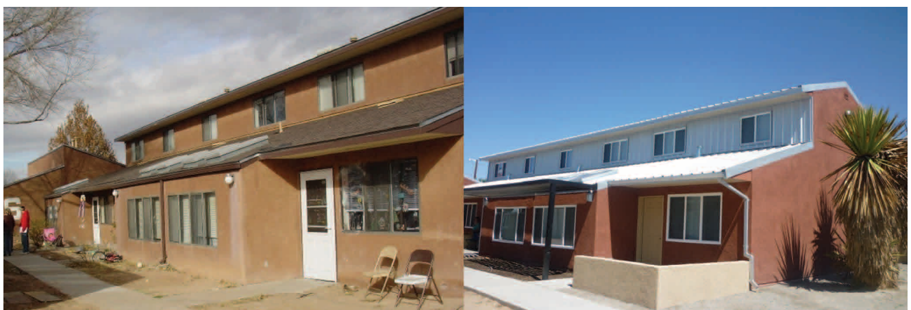
Belen Crossing in Belen, New Mexico, was overhauled using Low Income Housing Tax Credits.
