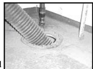
Temporary ventilation tube is routed through a butter-worth hole minimizing interference with access and egress
