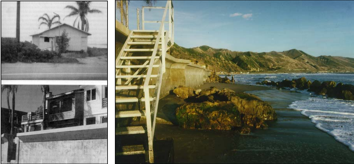
The Nollan Property. 1. The original structure on the Nollan property as viewed from the road. 2. The property built out as viewed from the beach. 3. A view of the beach, presumably from below the mean high tide line.
