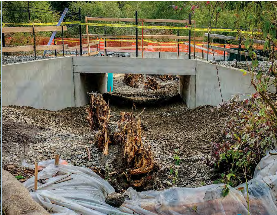
Restoring fish passage, Zackuse Creek culvert replacement (before and after)
