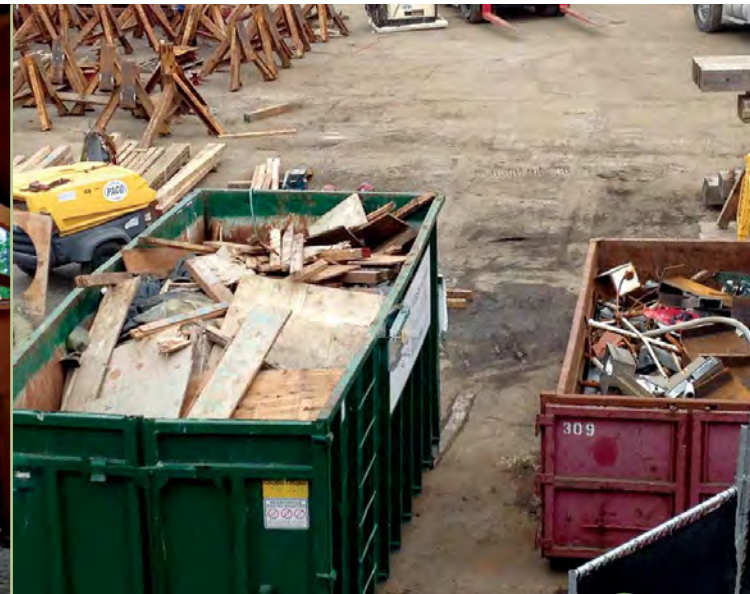
Source-separated recycling at the Colman Dock project in the City of Seattle.
