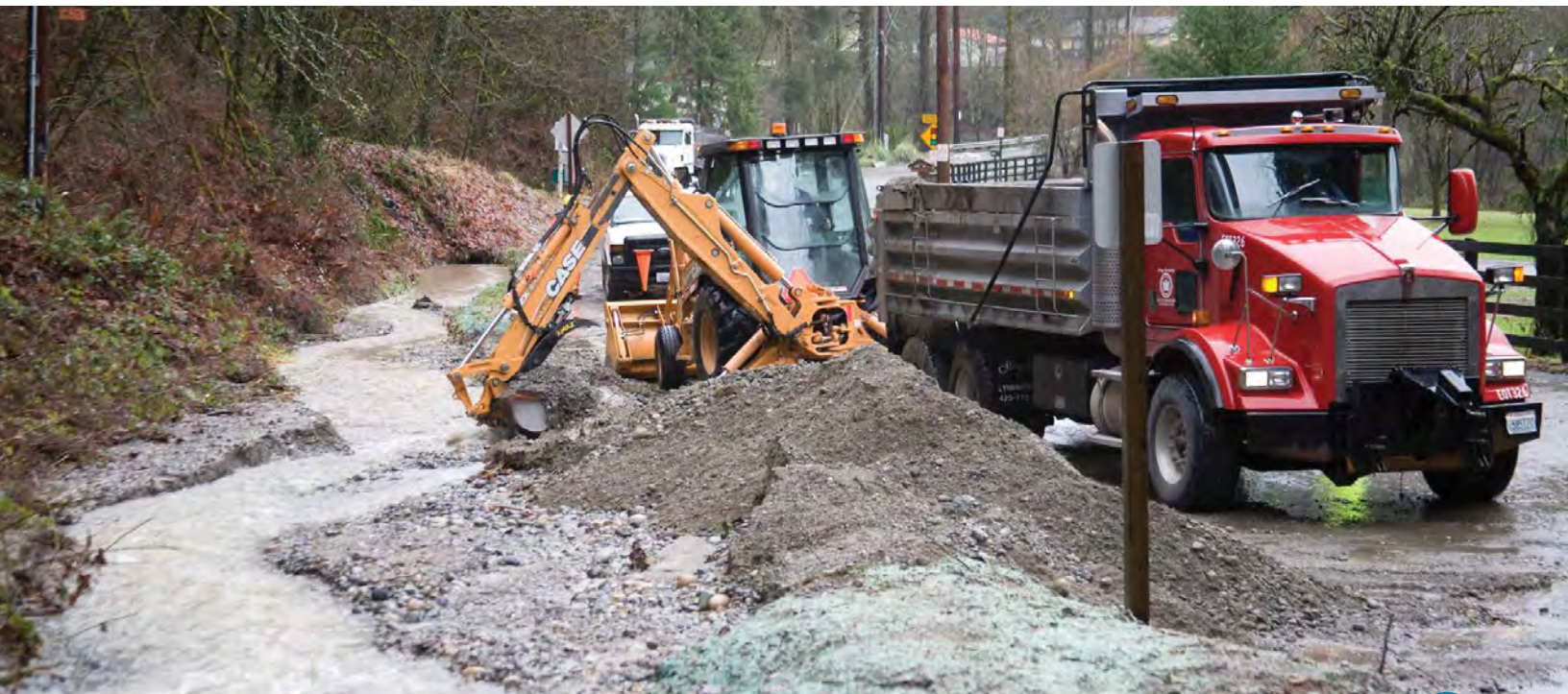
Clearing a landslide from Jones Road (2009)
