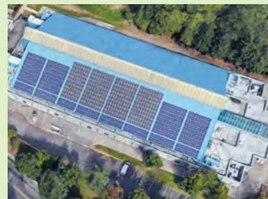
Weyerhaeuser King County Aquatic and Conference Center: 240,000 kWh/yr
