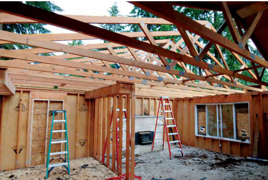
Deconstruction project at a site in Bellevue.
