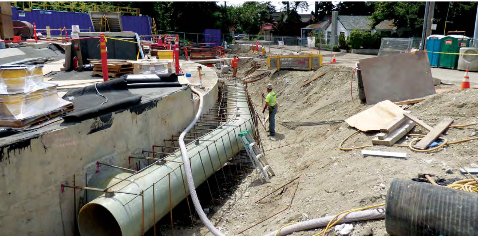
Murray Combined Sewer Overflow Storage Facility construction
