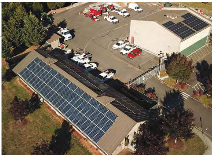
King County Parks' North Utility Crew Shop is the County's first certified net-zero energy project. The solar panels, installed on two buildings built over a decade ago, generate 40% more power than the site consumes each year.
