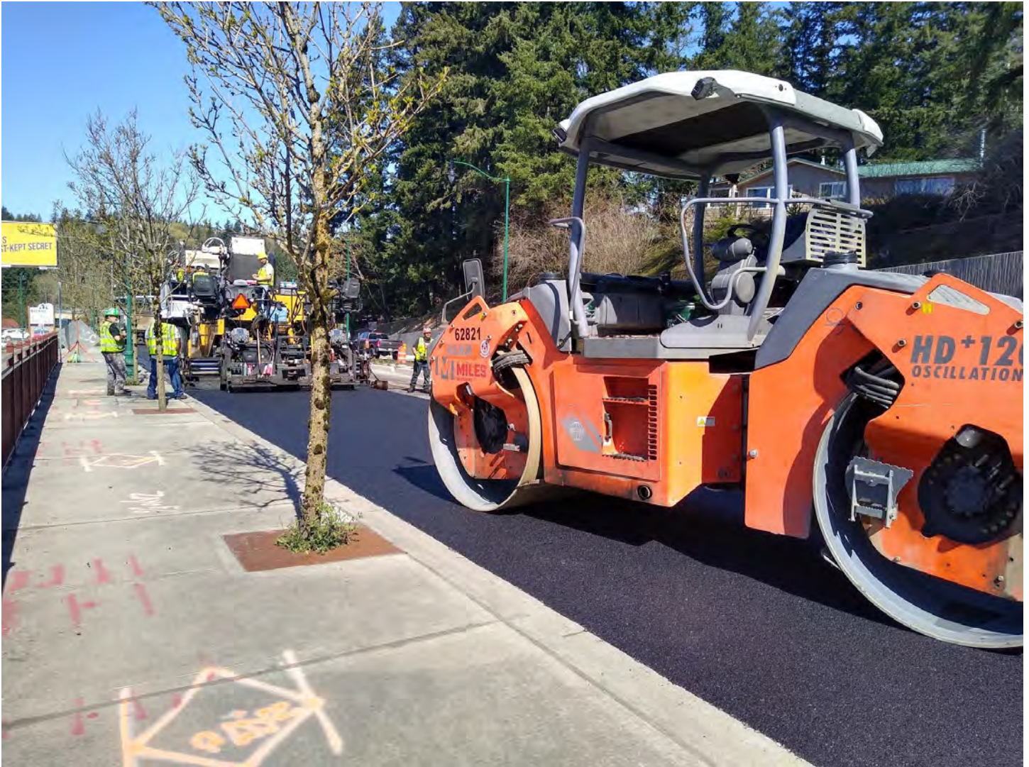
Road paving along HWY 169, Maple Valley
