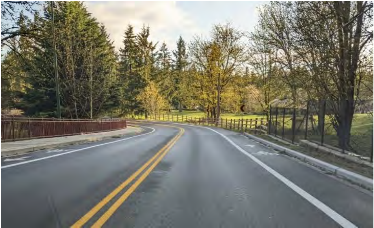
Fresh pavement and striping, Witte Road
