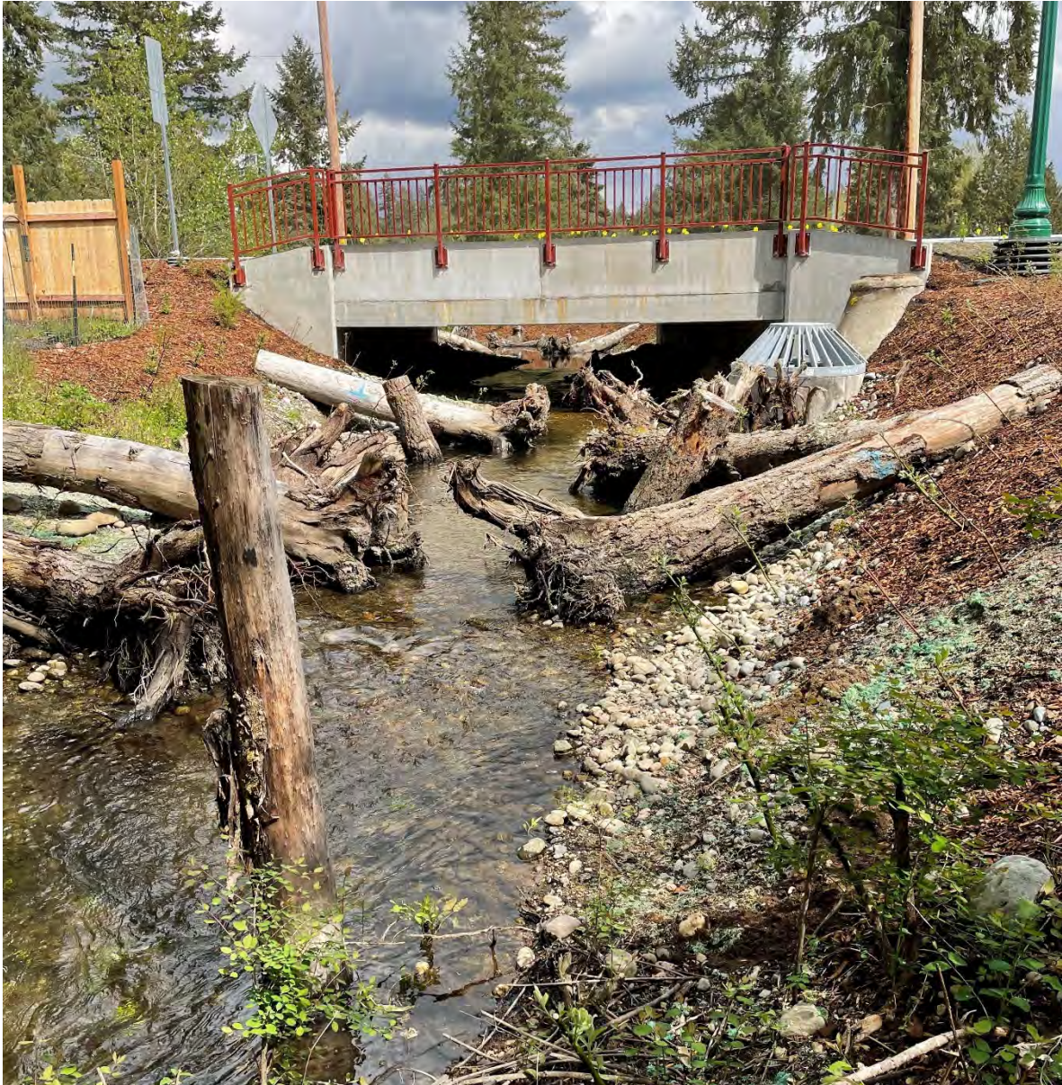
Jenkins Creek Culvert, Witte Road
