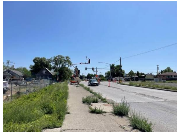
View of North Haven Street Facing South
